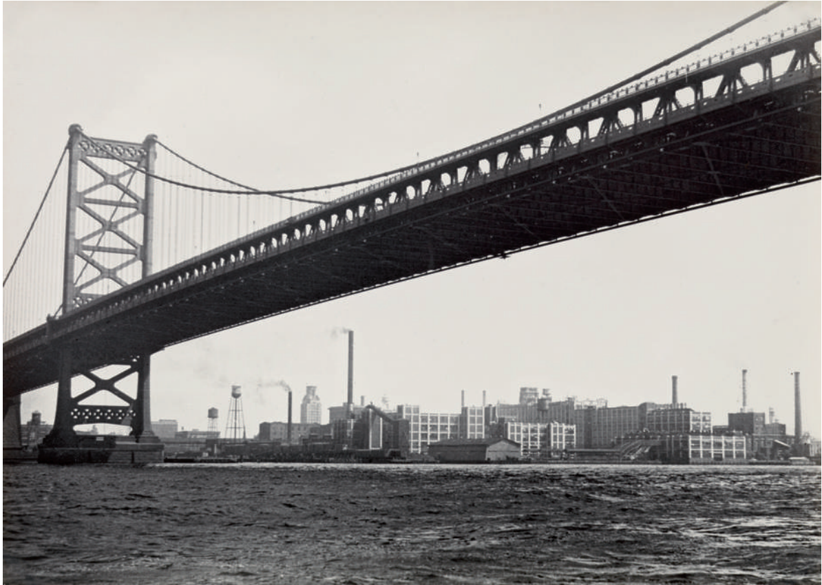
UMBO (1902–1980) Delaware Bridge, Philadelphia. 1952.
